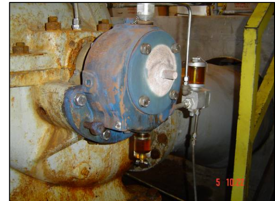
Sludge cup clean after 6 months operation
